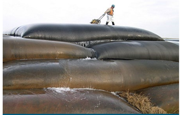
Geotubes Used for Dewatering at Onondaga Pond, NY.
