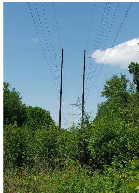
Typical proposed double monopole type structure
