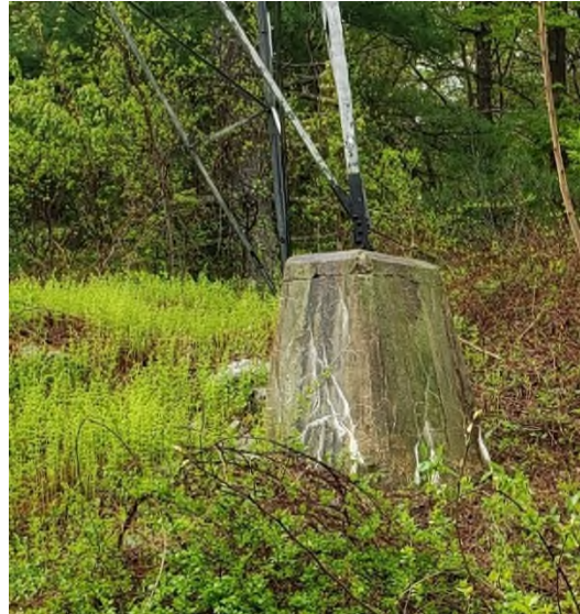
Typical lattice structure footing
