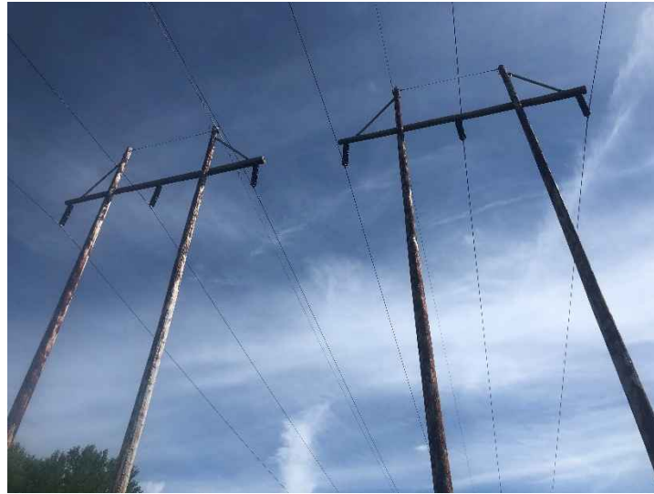
Double wooden H-frame Structure 10269 in Granby
