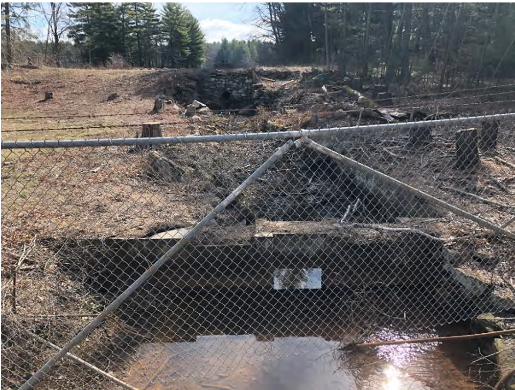
Photo 16 – Downstream overview of the dike from School Street
