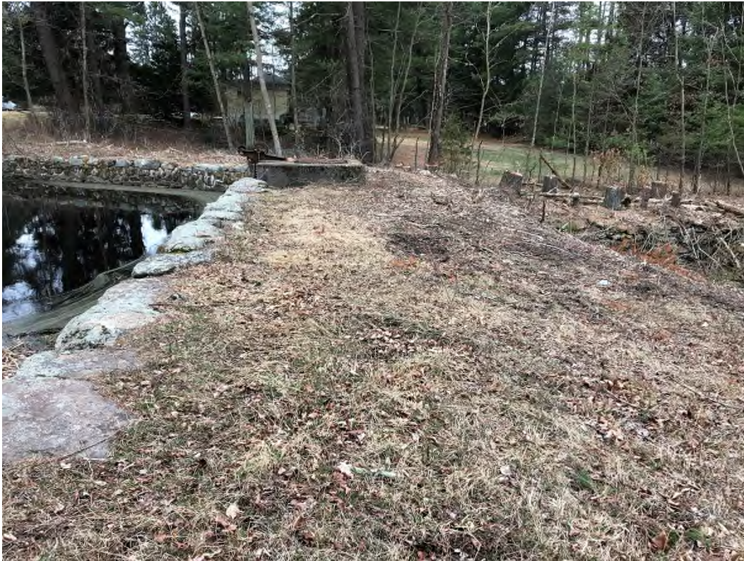
Photo 3 – Dike crest viewed from right end
