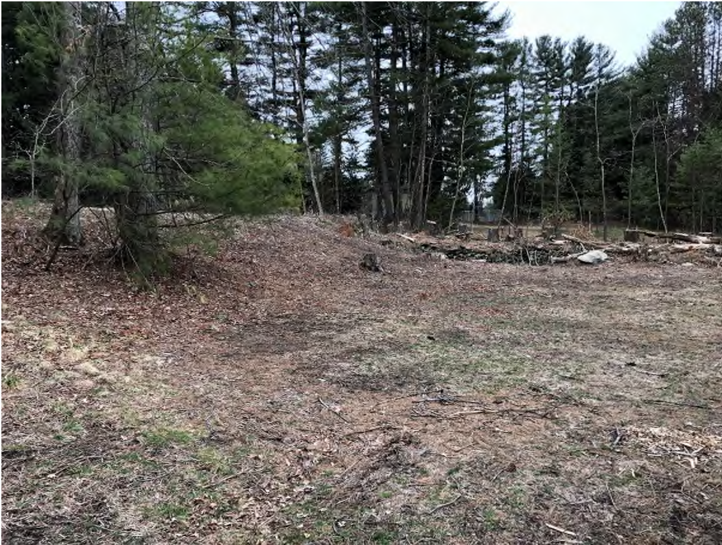
Photo 17 – Downstream overview of the dike from the right side
