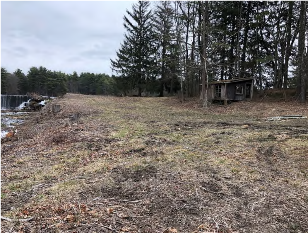
Photo 1 – Downstream view of embankment left of spillway
