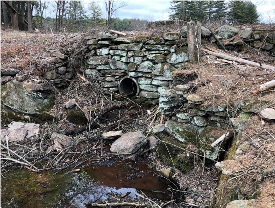
Photo 11 – Downstream stone masonry retaining wall at low level outlet
