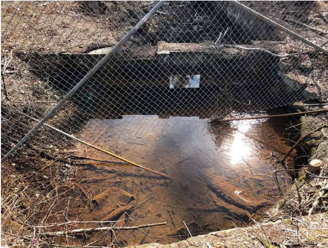
Photo 19 – Concrete weir in discharge channel downstream of the low-level outlet
