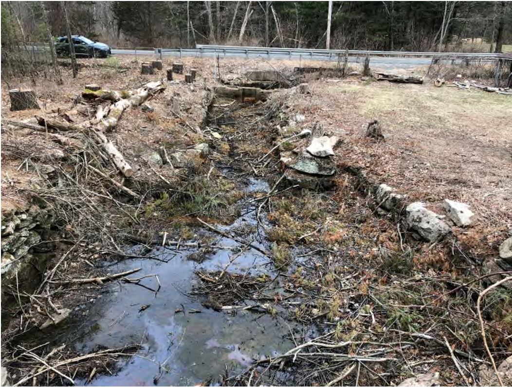
Photo 15 – Discharge channel viewed from the top of dike
