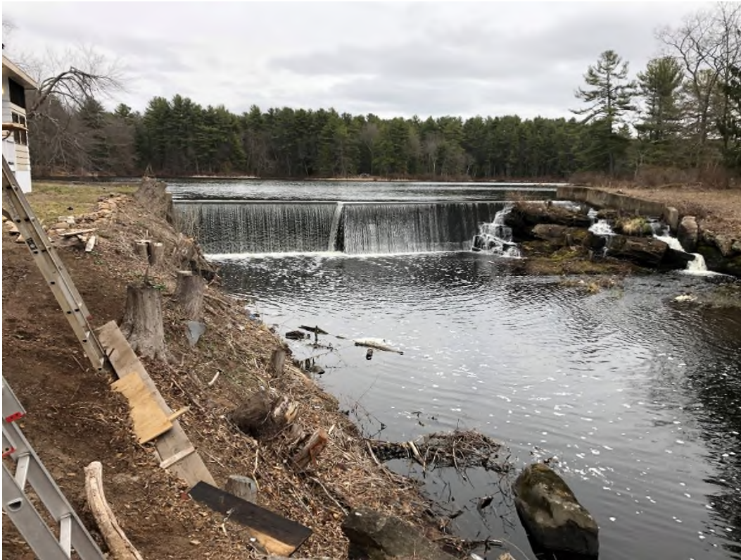
Photo 15 – Downstream view of spillway from right side
