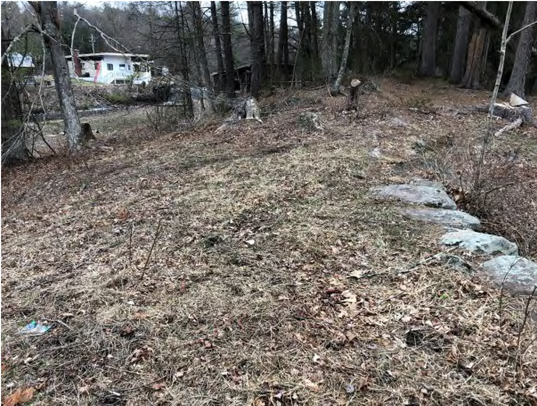
Photo 9 – Embankment crest at right abutment
