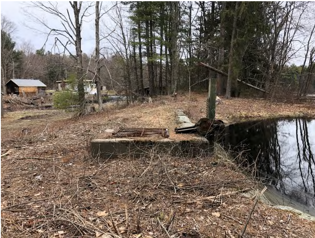
Photo 8 – Crest and low-level control structure viewed from the left side
