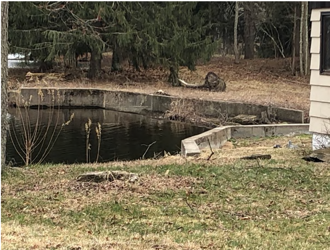
Photo 6 – Spillway and right training wall viewed from right side
