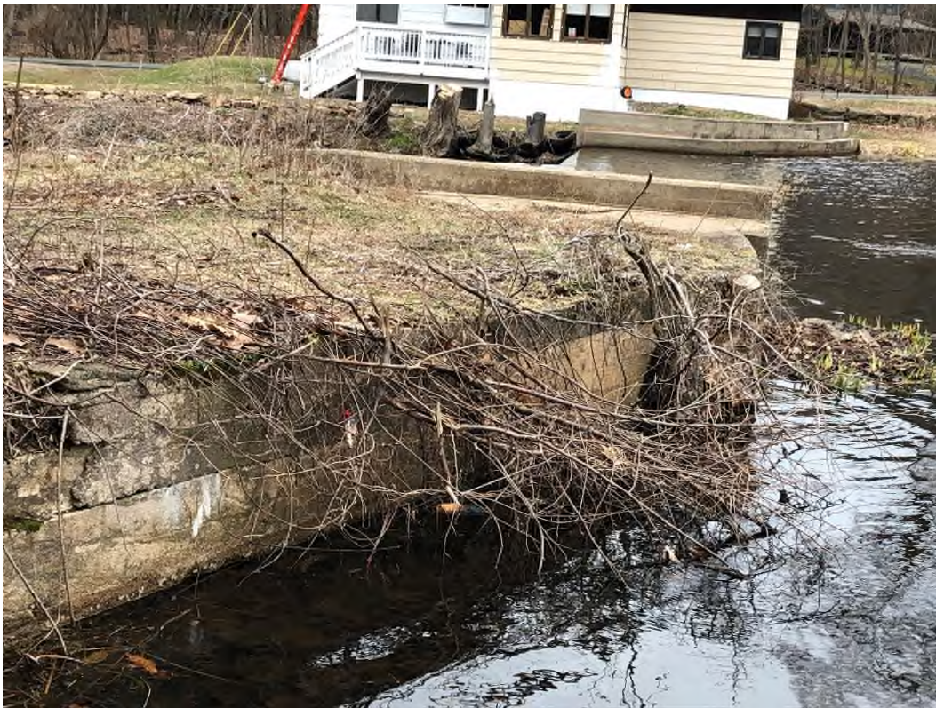
Photo 19 – Upstream left retaining wall
