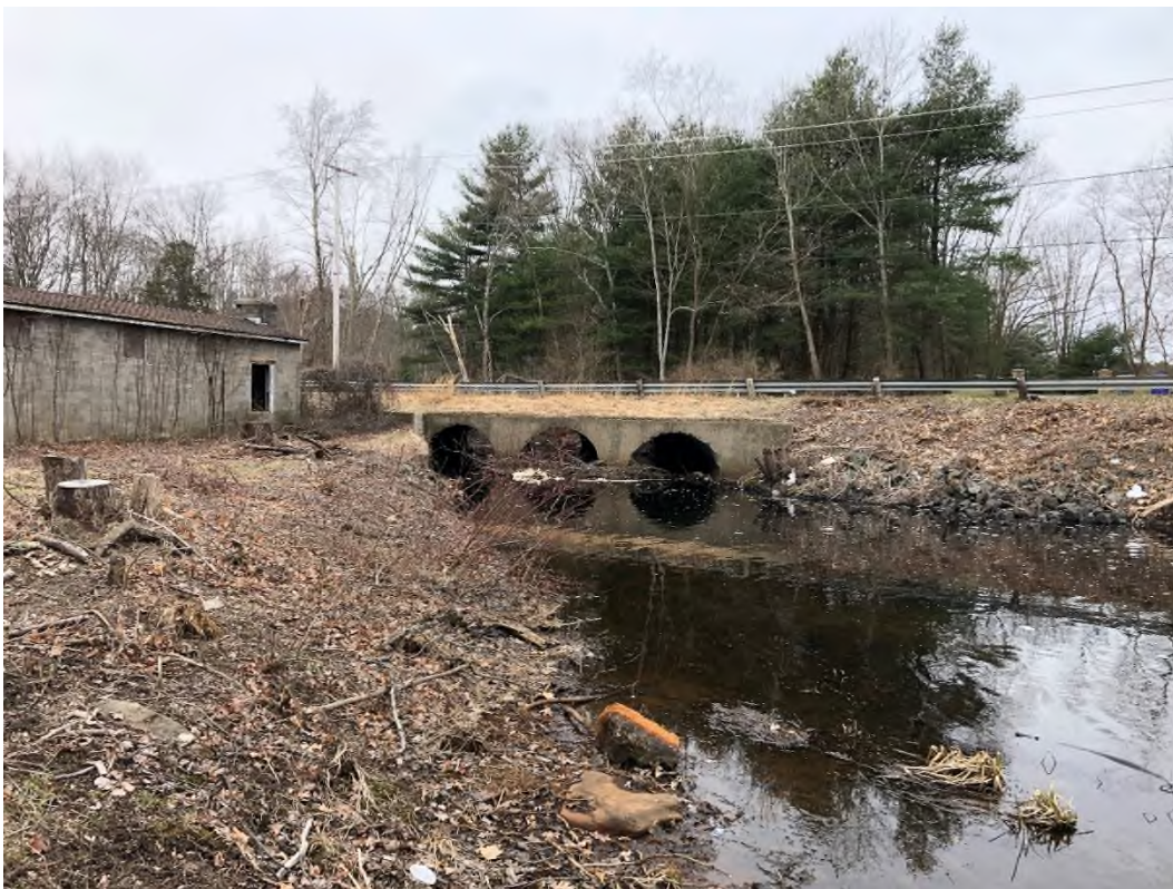
Photo 20 – Upstream view of ACCMP culverts passing under School Street downstream
