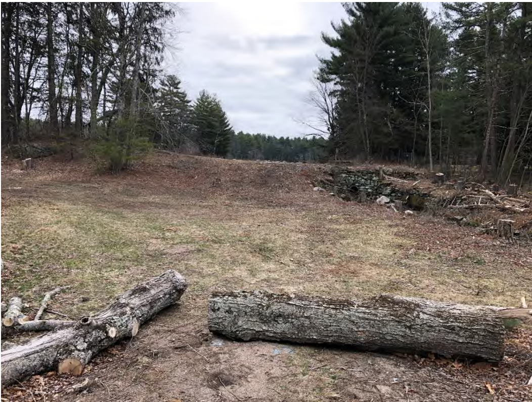
Photo 10 – Downstream slope at right side of dike
