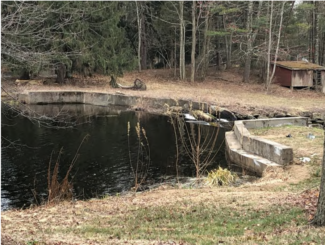
Photo 5 – Upstream overview from right side
