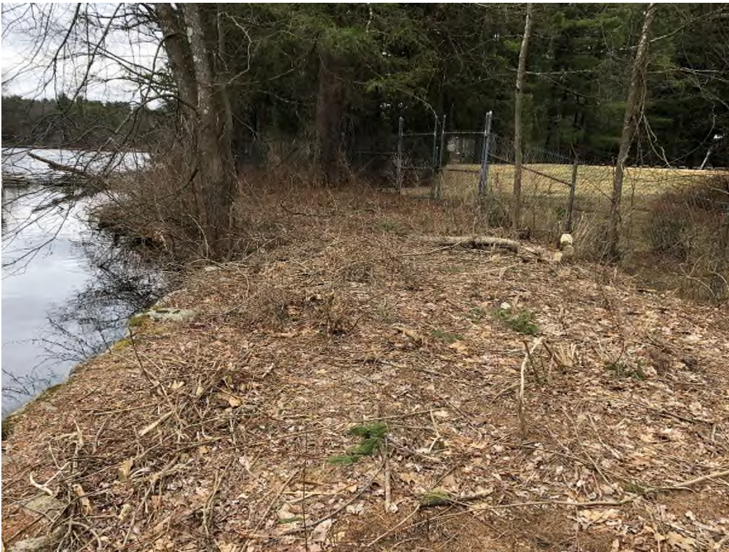
Photo 6 – Crest and view of left abutment
