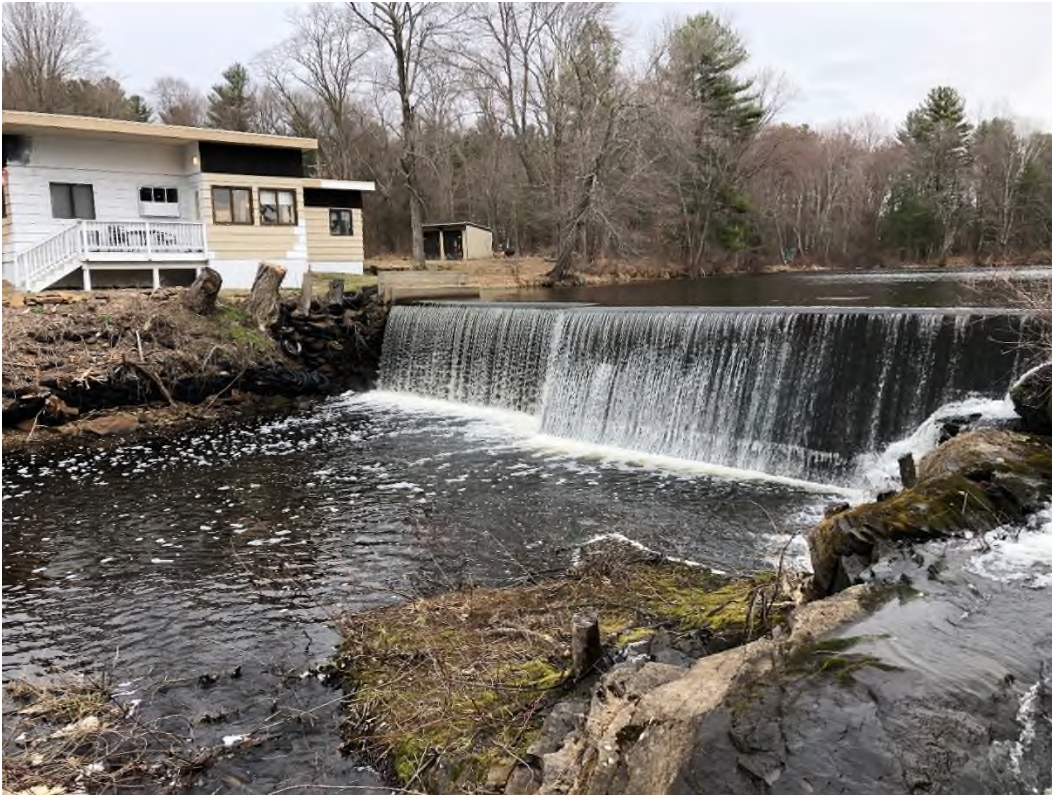
Photo 13 – Downstream side of spillway viewed from left side
