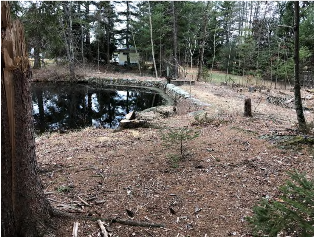
Photo 1 – Overview of upstream face of dike from right abutment
