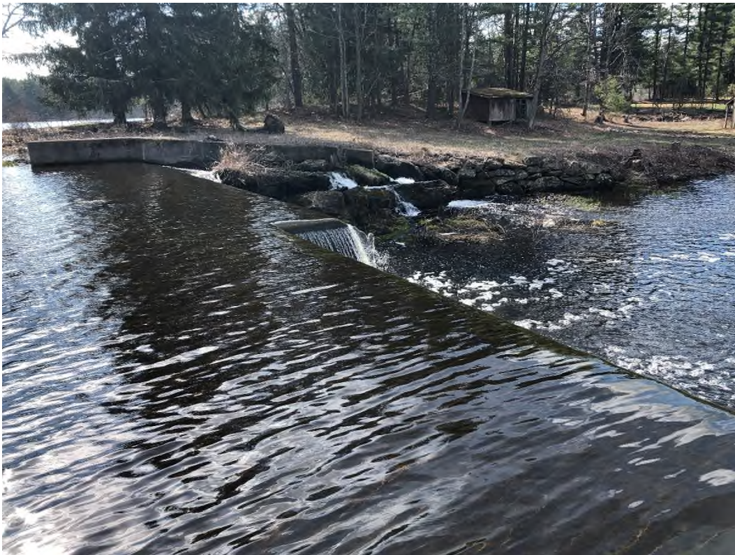
Photo 10 – View of jogged spillway crest and downstream area
