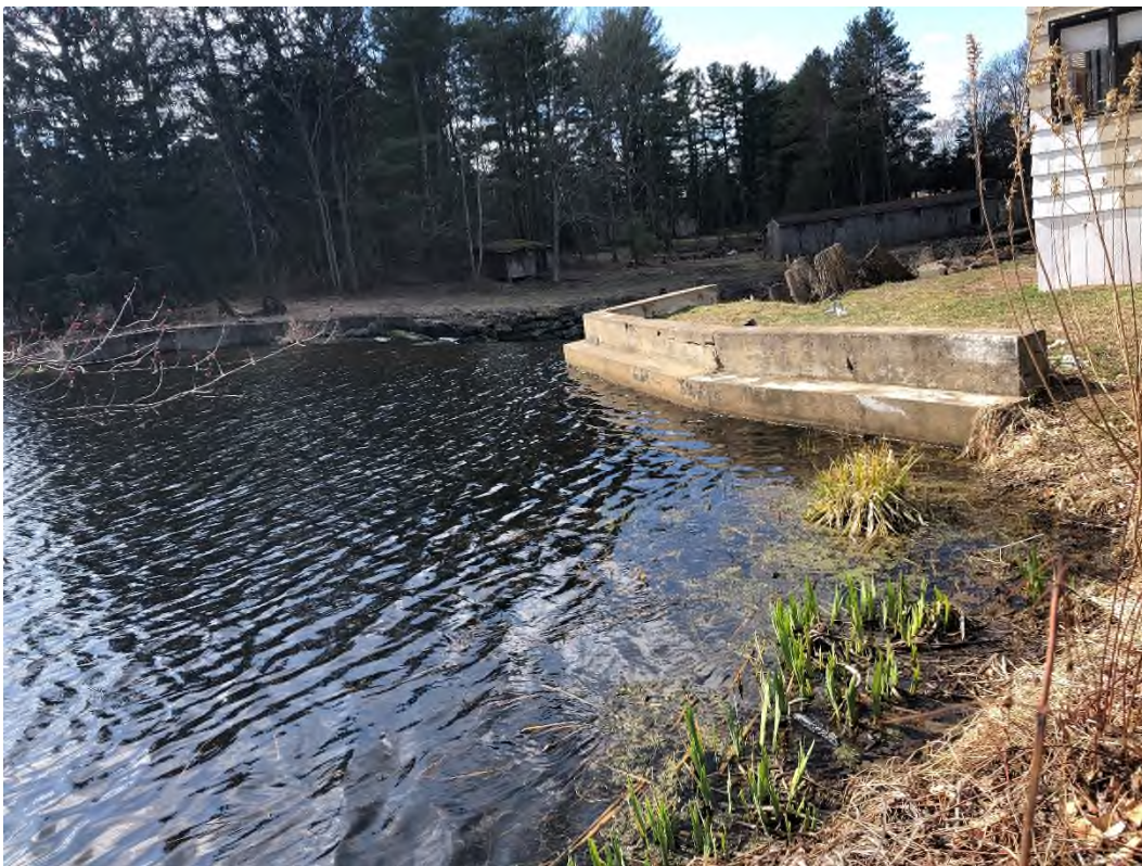
Photo 18 –Upstream face of right spillway training wall
