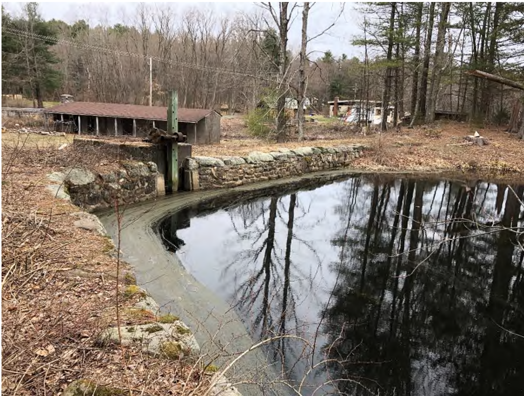
Photo 4 – Upstream face of dike from left abutment
