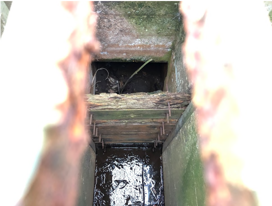
Photo 18 – Interior of low-level outlet structure looking downstream
