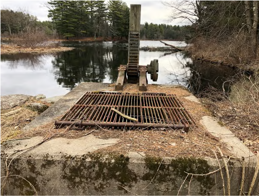
Photo 5 – Control gate structure viewed from downstream side looking into impoundment
