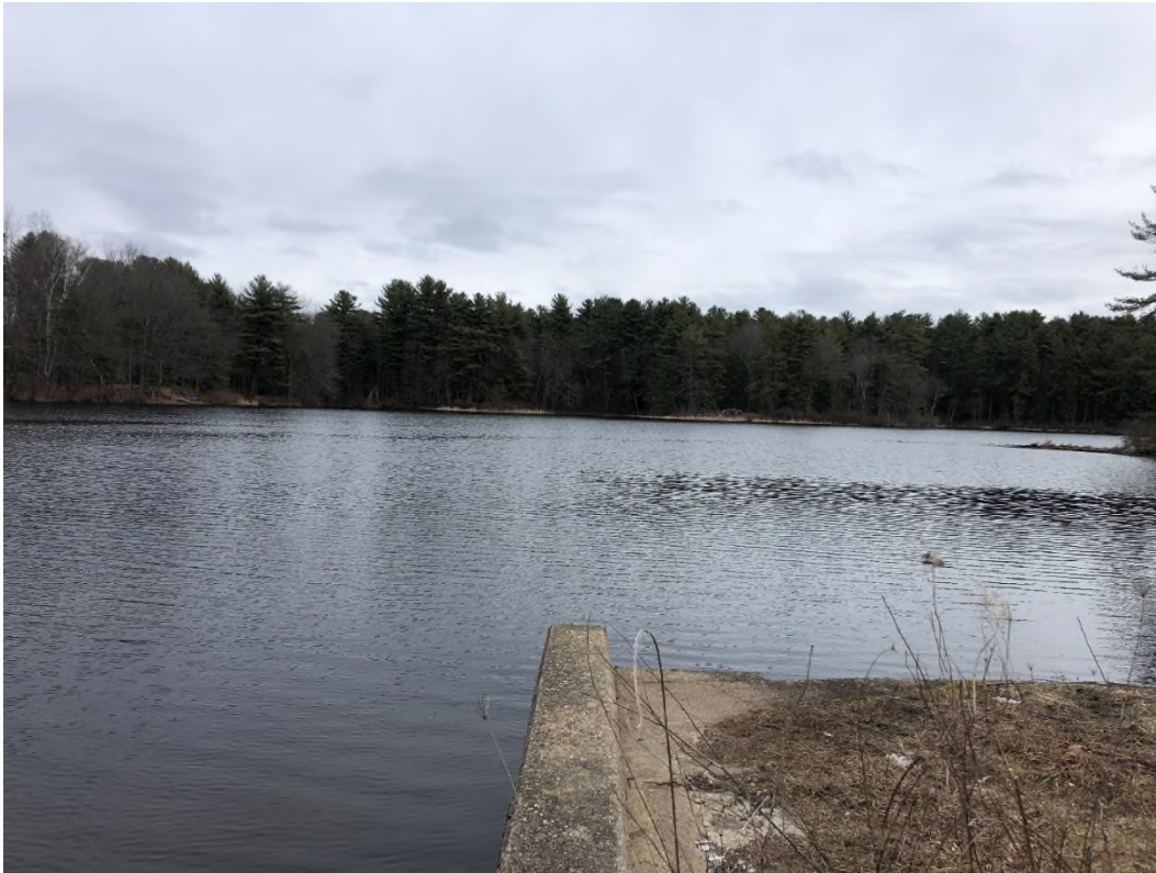
Photo 9 – View of impoundment and left upstream spillway training wall
