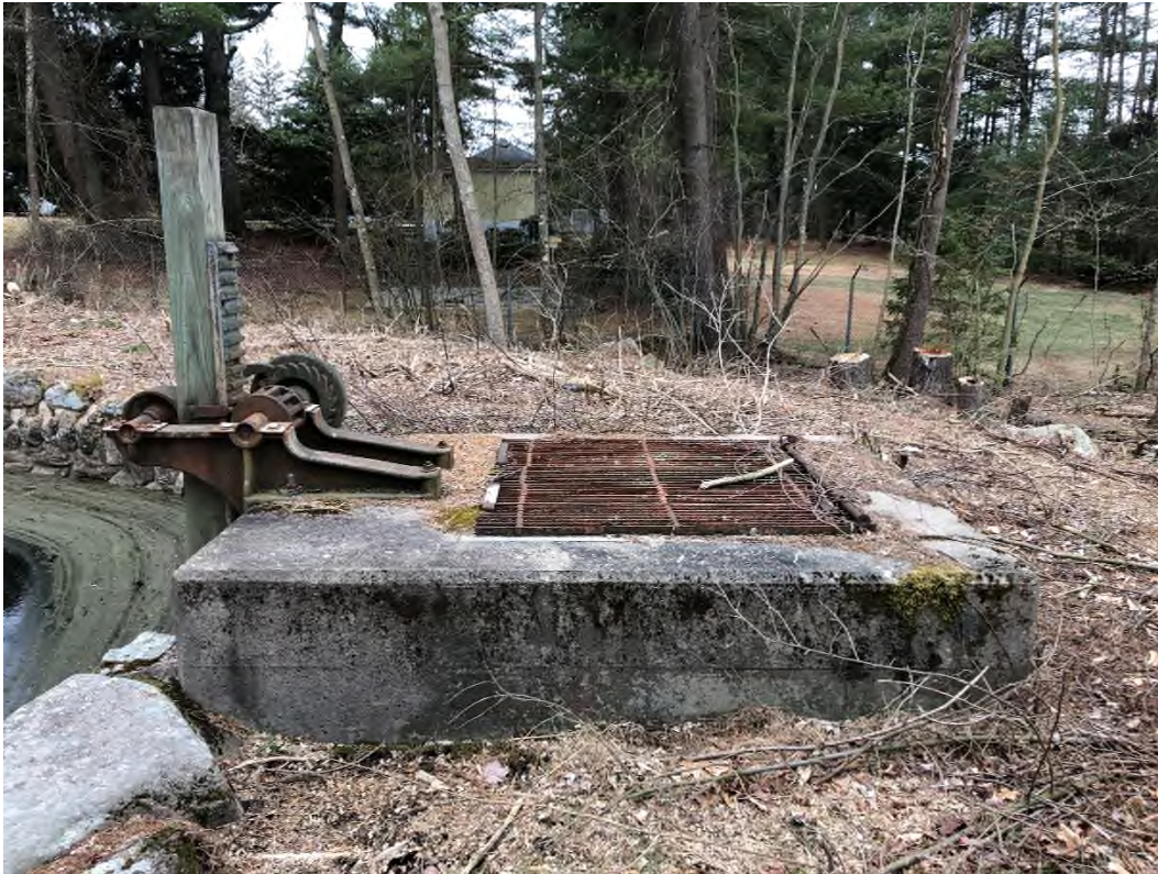
Photo 7 – Right side of rack and pinion level control gate structure
