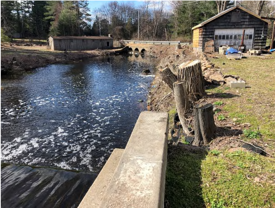
Photo 11 – Right upstream training wall and tree stumps downstream of spillway at right abutment.
