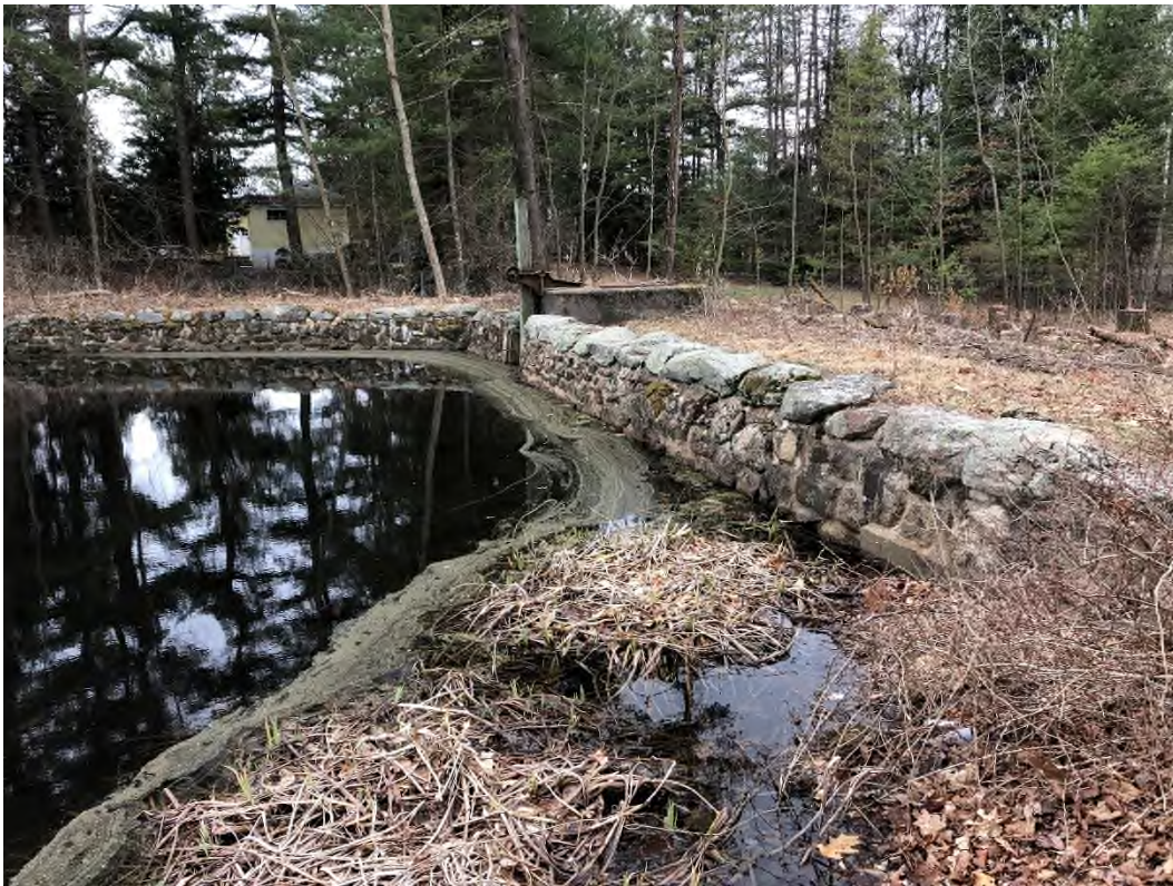
Photo 2 – Upstream face viewed from right end of dike
