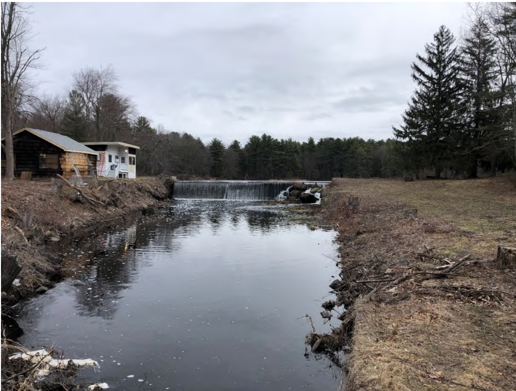
Photo 2 – Downstream overview of dam
