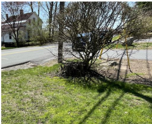
Image 1: Existing conditions at catch basin on Center Street during field assessment. Note the erosion at edge of road caused by stormwater flowing to catch basin.
