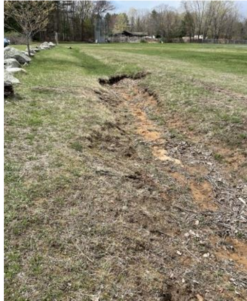
Image 1: The existing swale to be retrofitted. Note the upstream extent of severe erosion in the existing swale, with exposed soils visible where erosion has already occurred.
