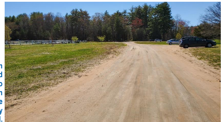
Image 1: The existing swale to be retrofitted. Note the upstream extent of severe erosion in the existing swale, with exposed soils visible where erosion has already occurred.
