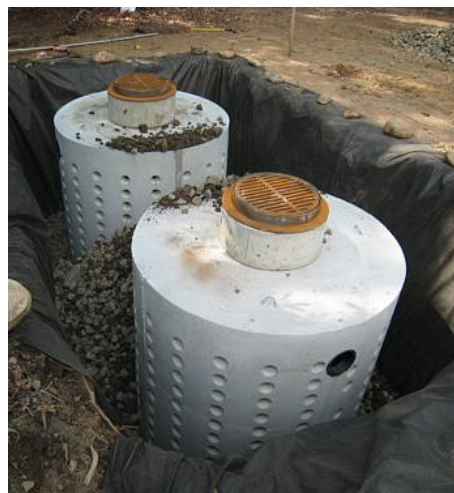
Image 1: Typical infiltrating catch basin installation.
