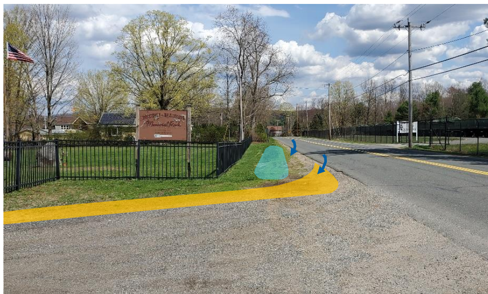
Image 3: Location of the proposed bioretention swale (blue) in the right-of-way east of the entrance to Brown Ellison Park. Restoration of grass ground cover and placement of boulders is recommended (orange) along both sides of the driveway.
