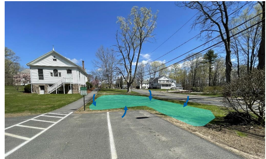
Image 3: Proposed L-shaped bioretention basin.
